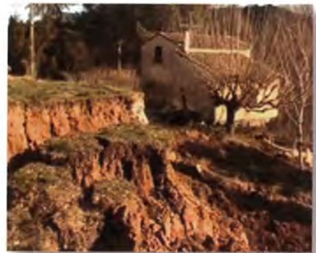
Habitation concernée © France 3
